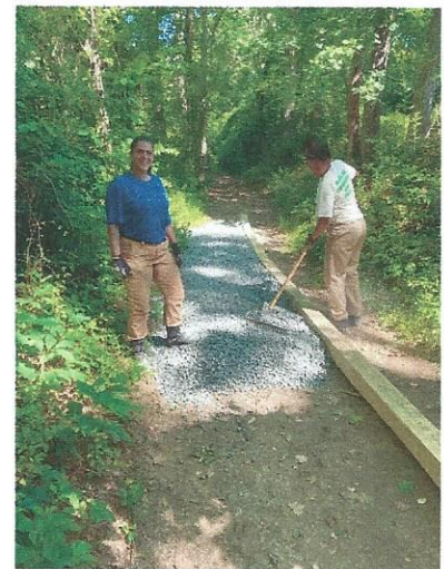
CJC Trail Maintenance, 2021
