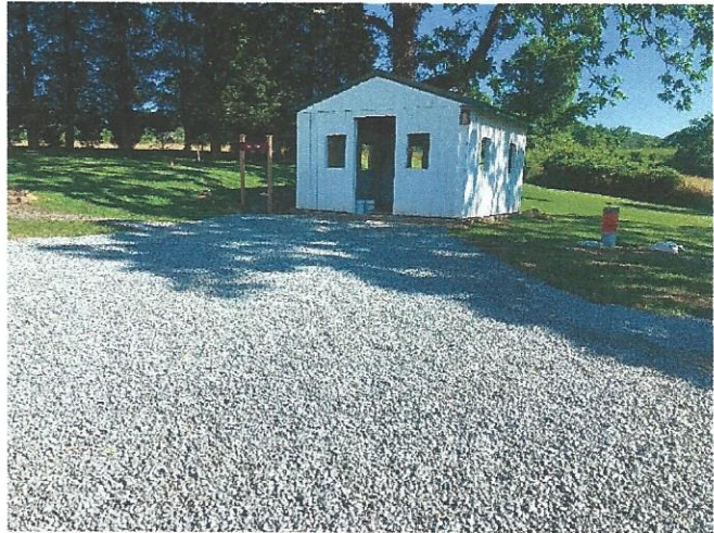
Drainage repairs at the chicken coop.
