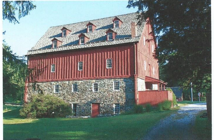
Grist mill south wall - 2015
