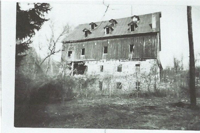
Grist mill south wall – 1985
